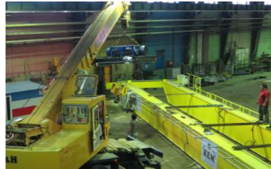
Crane Rails installation Service
