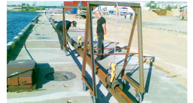
Rails Maintenance Service
